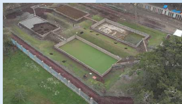
The rehabilitated constructed wetland Amora Gedel.
