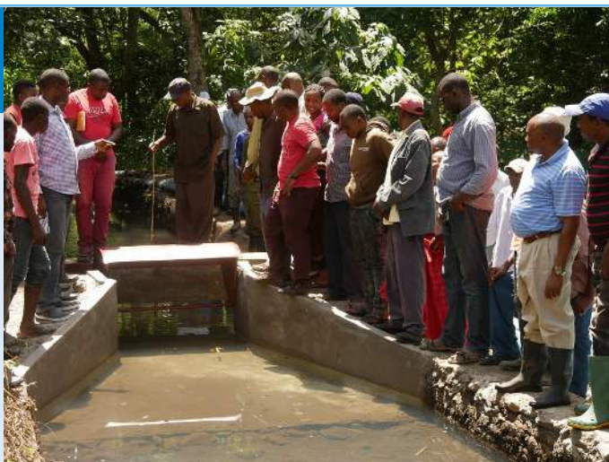
Partners visiting a reconstructed furrow distribution gate.
