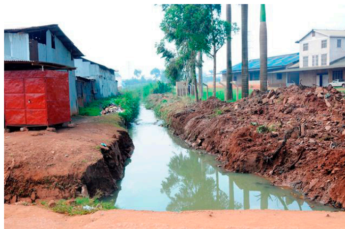
Desilting and waste collection at drainage channels in Nalukolongo.
