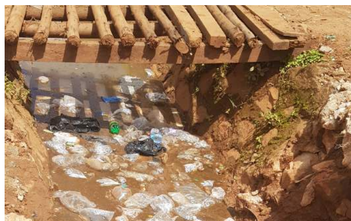
Pollution of waterways in Greater Kampala with plastic waste. Improperly disposed plastic waste causes blockage of drainage systems and increases the risk of flooding.
